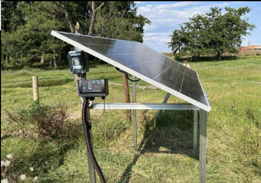
Solar-Powered Well-Point System with Automated Micro-Nebulisers to secure topsoil moisture for standing freshwater habitats
